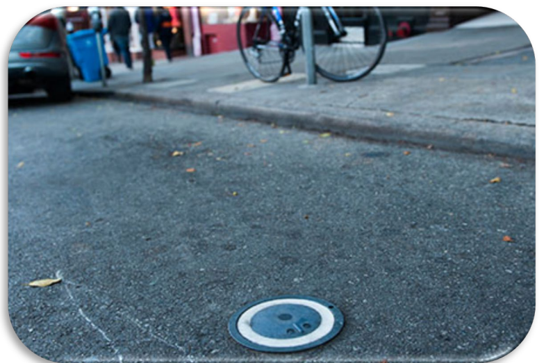
Figure 68. An in-ground parking sensor installed on a public parking space.
