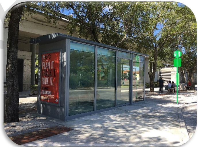
Figure 95. Air-conditioned Bus Stop at Hialeah Metrorail Station
