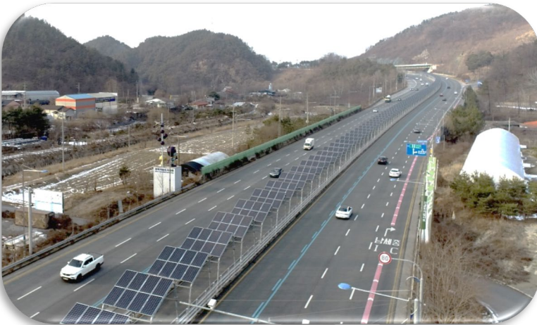
Figure 85. South Korea's solar-powered bike path.
