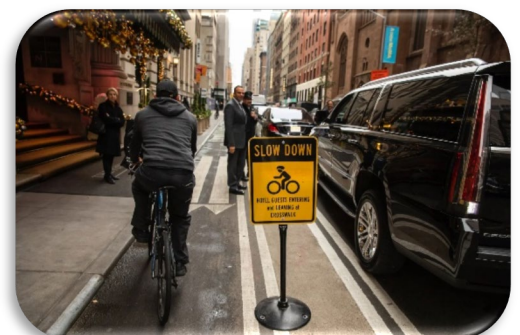
Figure 64. NYC bicycle lane equipped with rumble strips, enhanced pavement markings, and signage.
