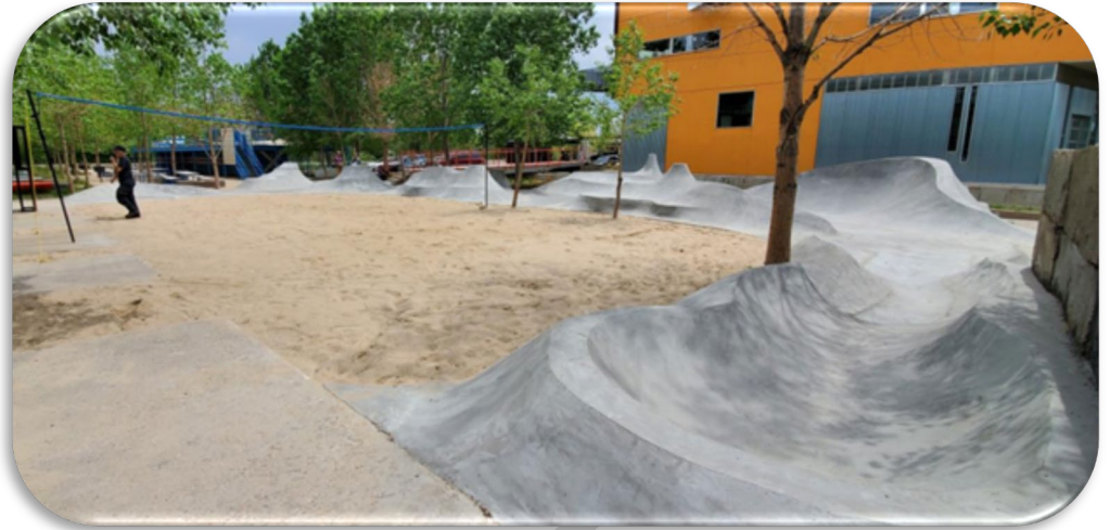
Figure 84. Skate park facility redirects stormwater to collection areas
